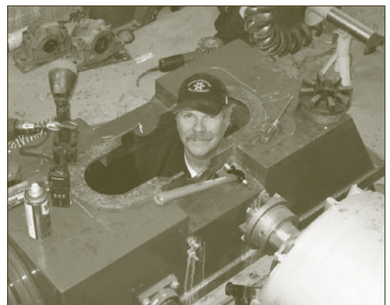
The Snowmass hydroelectric plant generates $10,000 of clean energy each summer. Frank White runs the system.
